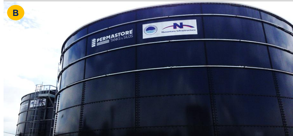
(B) New Reservoir Tanks (2 x 3,000 m 3 )
