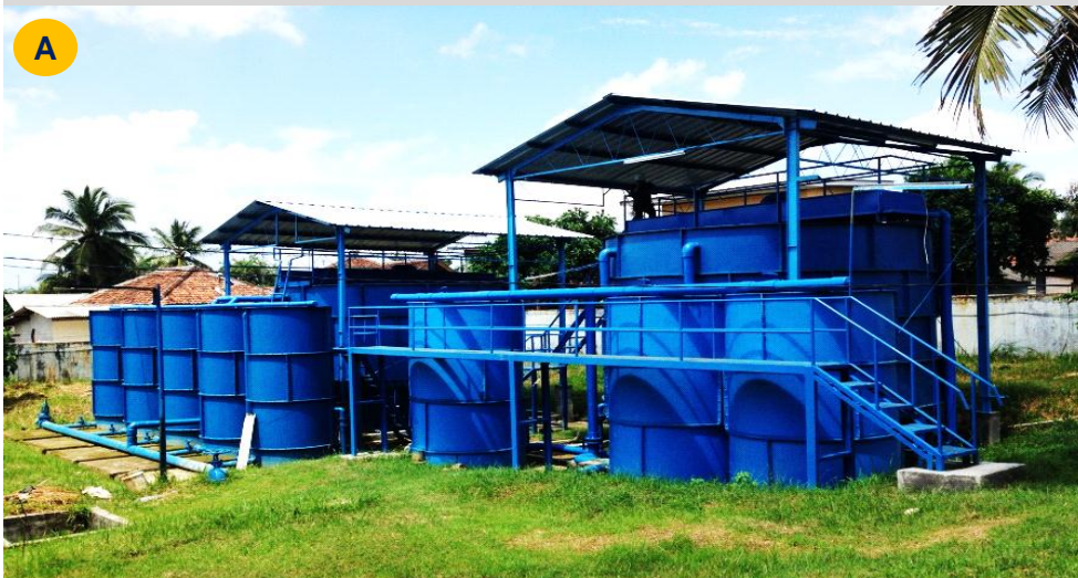
(A) Water Treatment Plant 1 & 2: Capacity 2 x 50 lps (Total 100 lps)
