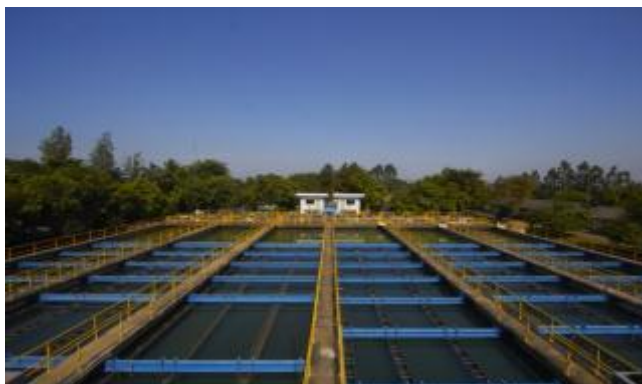
6 NOS Sedimentation Tanks
